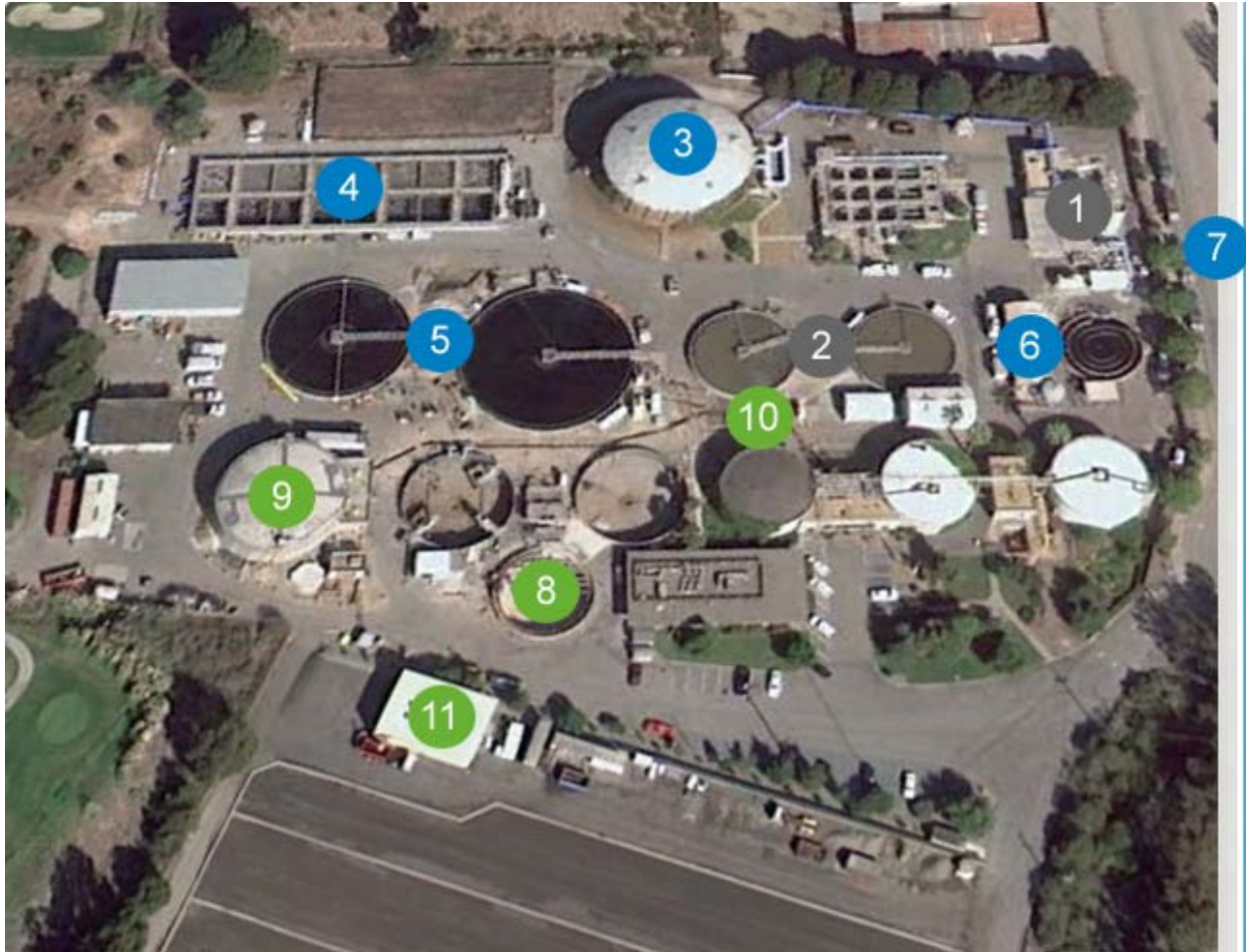
Figure 1.2.1 -- Aerial View of the San Leandro WWTF
